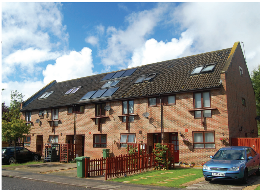
The discreet roof-integrated Clearline solar panels are the only outward indication that this house is 80% more energy efficient than its neighbours.
